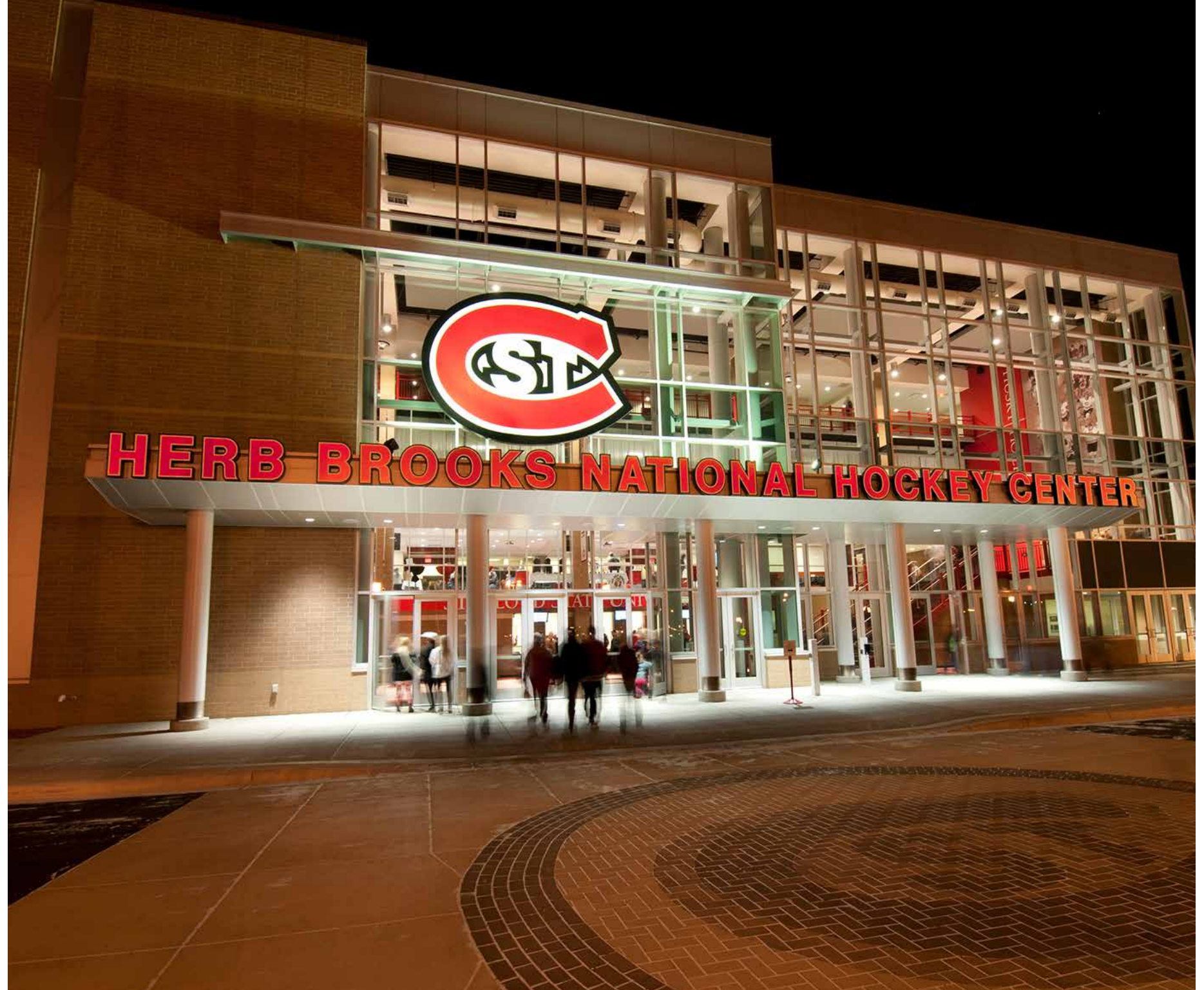
HERB BROOKS NATIONAL HOCKEY CENTER RENOVATION St. Cloud State University | St. Cloud, Minnesota
