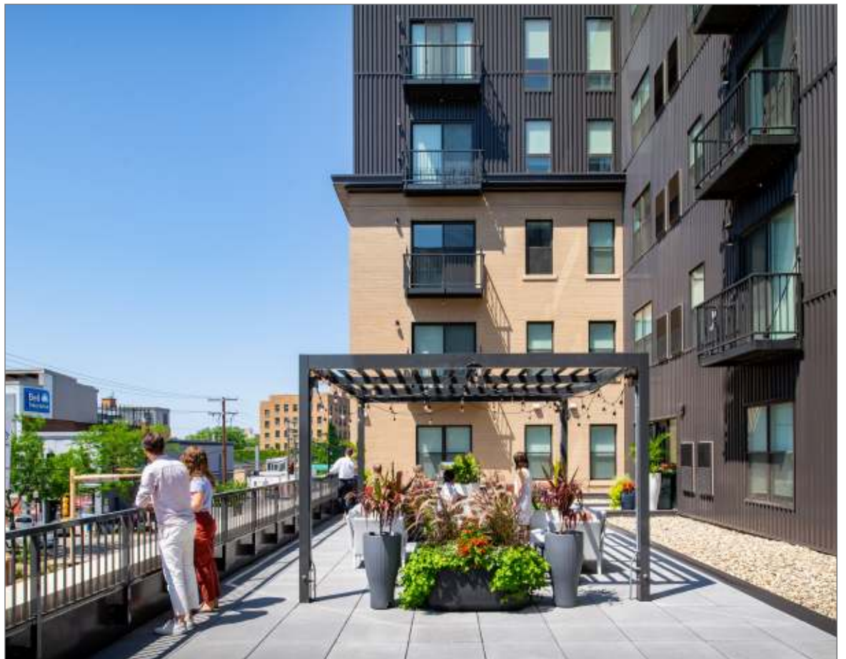
JLG Architects' Mercantile project in Fargo, N.D., pays tribute to the building that formerly stood on the site through traditional masonry, patterns, and the scale of the facade, according to the firm. (Photo credit: Chad Ziemendorf)
