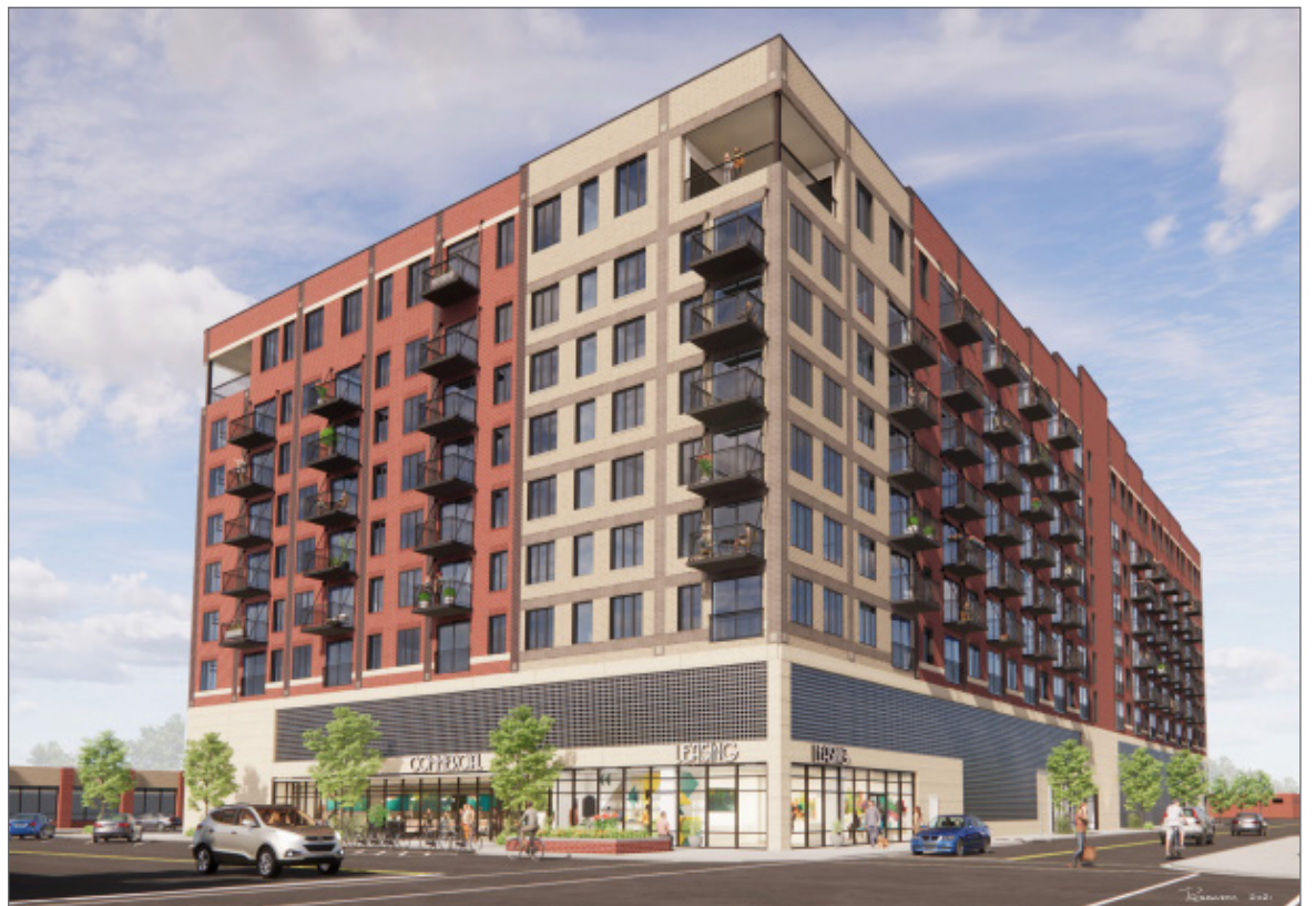
Rosemann & Associates designed Oxbow for Sunflower Development Group. The 208-unit project, located in Kansas City, Mo., was constructed on 1.4 acres and includes 3,500 square feet of first-floor retail. The project includes one- and two-bedroom floor plans as well as penthouse suites.
